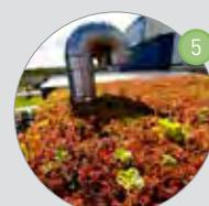
The green roof reduces heat loads and can also process parts of the grey water produced in the unit
